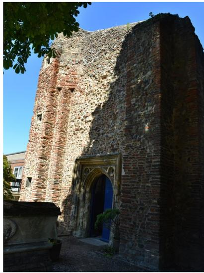
Notice the re-used Roman bricks that were used in the building of St Martin's tower in Saxon (Orthodox) times, and in its repair since the Civil War, after it was hit by cannon fire in the siege of Colchester in 1648, but never completely rebuilt.
